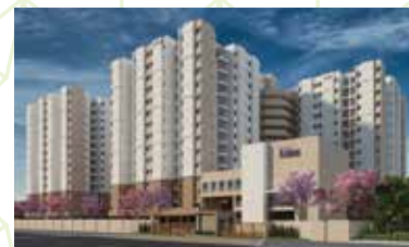
ASHRAYA Bengaluru - Mysuru Expressway, Bidadi
