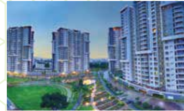
GREENAGE Hosur Main Road, Bengaluru
